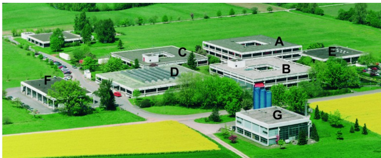
760 Fig. 2: New Institute Buildings. A: first floor: Library, Administration, Lecture Hall, second and third floor: scientists' studies, B: first floor: drawing and documentation, computer center, test facilities, clean rooms, first floor: scientists' and engineers studies. C: Electronic workshop, D: mechanical workshop, mechanical and electronic supply, E: Cafeteria and meeting rooms, F: Garage, G: Power plant. (Source: MP Ae)
