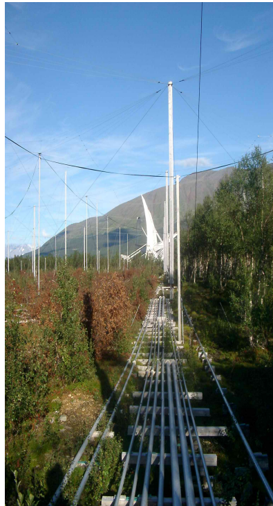
775 Fig. 7: Detail of one of the HEATING antenna arrays. The aluminium pipes on the ground serve as co-axial cables to feed the power to the dipoles. In the background the EISCAT VHF antenna is visible (Source: M.T. Rietveld).
