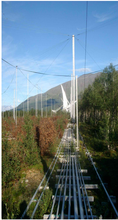
Fig. 7: Detail of one of the HEATING antenna arrays. The aluminium pipes on the ground serve as co-axial cables to feed the power to the dipoles. In the background the EISCAT VHF antenna is visible (Source: M.T. Rietveld).
