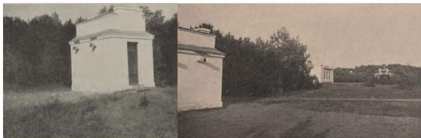
Figure 2. House built for atmospheric electricity measurements at Świder. Left: Side view of the building as shown in Kalinowski (1932). Right: Side view with one magnetic building in the background, view from Zacisza Street, reproduced from Szpecht (1939), page 205. The open area next to the building is visible, as well as holes in the building for pulling wires through, on such wire is sketched in Fig. 5). A larger area for measurements in the open space spread further to the right – see also the photo in the left panel of Fig. 1.
