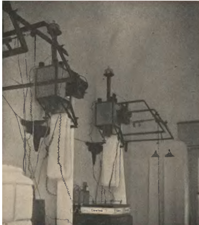
Figure 5. Inside of the atmospheric electricity measurement house with a view on the wall with two installed Benndorf electrometers. The electrometers are hanged on the wall. The casing of each electrometer is earthed, and its plate electrodes are connected to a battery standing on the floor. The electrometers' needles are connected to wires coming from the outside themselves connected to radioactive probes. Photograph from Szpecht (1939), page 214 (public domain).
