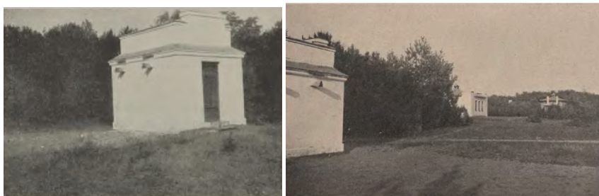
Figure 2. House built for atmospheric electricity measurements at Świder. Left: Side view of the building as shown in Kalinowski (1932). Right: Side view with one magnetic building in the background, view from Zacisza Street, reproduced from Szepecht (1939), page 205. The open area next to the building is visible, as well as holes in the building for pulling wires through, on such wire is sketched in Fig. 5). A larger area for measurements in the open space spread further to the right (see also the photo in the left panel of Fig. 1, and the diagram in Fig. 6).
