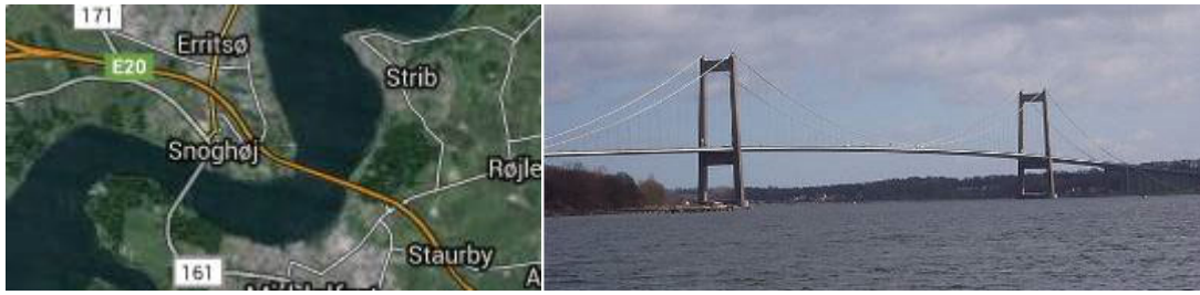
75 Figure 4. The highway bridge over Little Belt (© Google Maps and Wikipedia)
