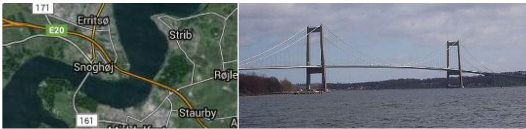
Figure 4. The highway bridge over Little Belt (© Google Maps and Wikipedia)
