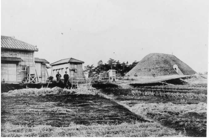
Figure 4: The 'Ishimuro' variation house (right) and the absolute hut (left). Ishimuro was used till 1980's (photo supplied by Kakioka Magnetic Observatory).
