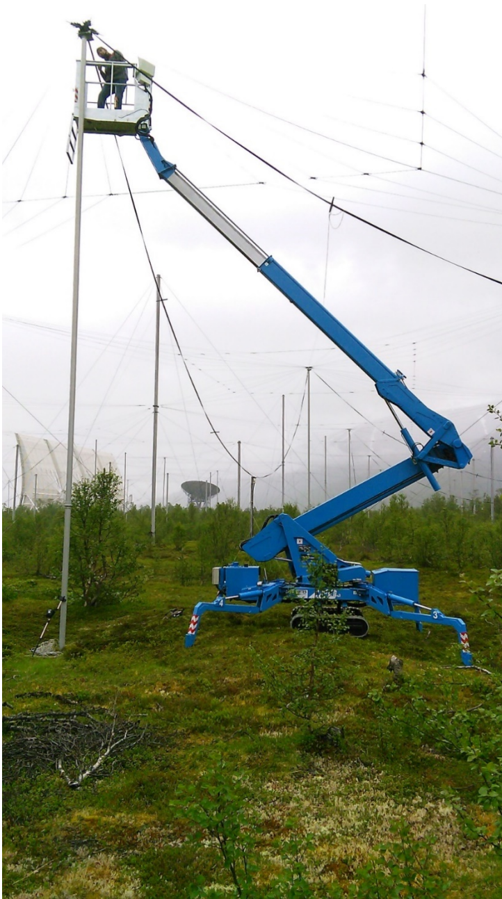
Figure 7: Repair work to one of the 12 m high antennas out of 144 such antennas in Array-1 to bypass existing and potential weak points in the twin-feed cable connection to the antenna centre. The original 23 m wooden masts are visible in the background. Note the different support mast and feed-lines compared to the original design as used in Arrays-2 and -3 shown in Fig. 3. (Photo M. T. Rietveld)
