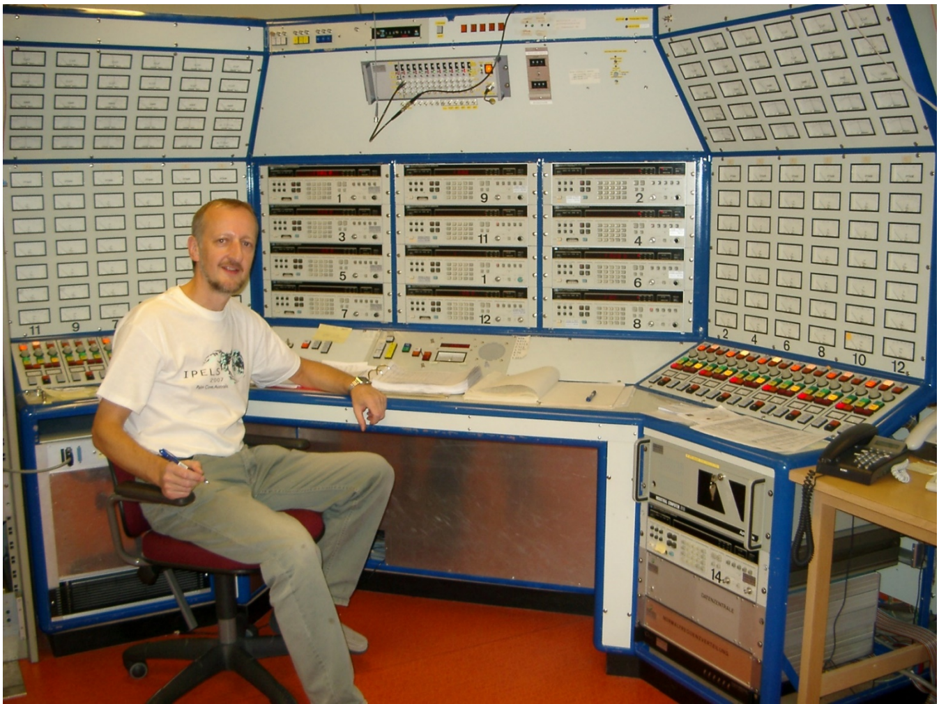
Figure 6: The heating facility console in the control room as it was in 2007, with the first author at the controls. Six columns of meters, lights and push buttons on each side show the status and are used to control each of the 12 transmitters. The twelve commercial RF synthesizers in the middle of the console have been replaced by digital synthesizers in the transmitter hall and the space is now filled by large computer screens. (Photo M. T. Rietveld).
