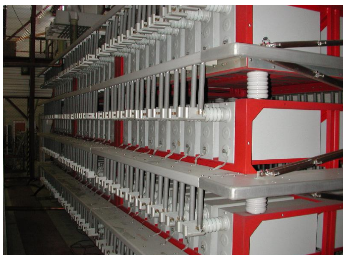
290 Figure 1: Left, an overview over part of the capacitor bank. Right, the "crowbar" spark gap. Photo courtesy of Ralf Larsen, Tromsø, formerly with EISCAT.
