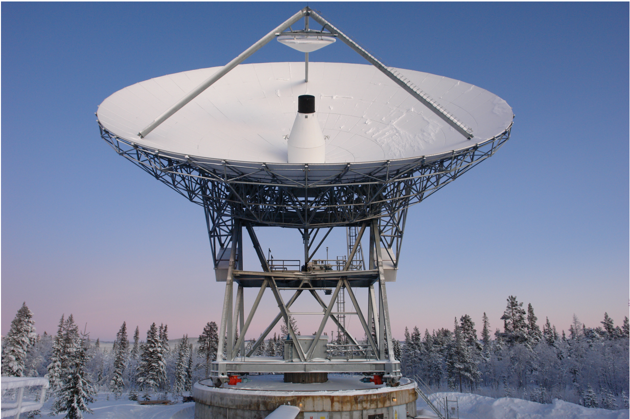
Figure 5: The Kiruna EISCAT UHF antenna. The Tromsø and Sodankylä antennas were identical, apart from the feed system of the Tromsø one, that included a waveguide run with rotary joints connecting to the transmitter. Photo courtesy of Lars-Göran Vanhainen, Swedish Institute of Space Physics (IRF).
