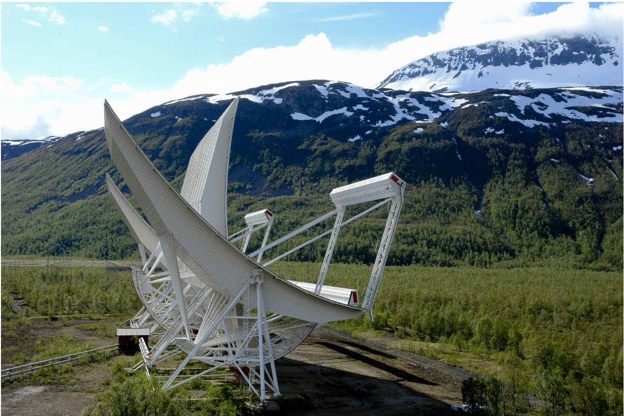
695 Figure 6: The EISCAT VHF parabolic cylinder antenna at Tromsø. It is constructed as four individually tiltable 30x40 m reflector / feedline segments, which however must be electrically operated either as a single 120x40 meter aperture (Mode 1) or as two independent 60x40 meter apertures (Mode 2). Photo courtesy of Lars-Göran Vanhainen, Swedish Institute of Space Physics (IRF).
