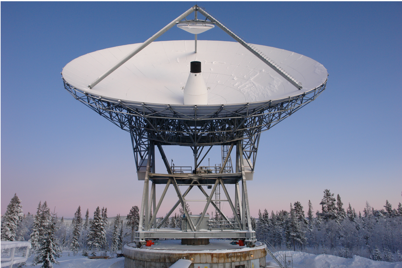
Figure 3: The Kiruna EISCAT UHF antenna. The Tromsø and Sodankylä antennas were identical, apart from the feed system of the Tromsø one, that included a waveguide run with rotary joints connecting to the transmitter. Photo courtesy of Lars-Göran Vanhainen, Swedish Institute of Space Physics (IRF).
