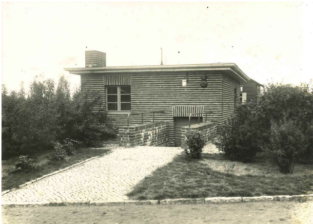
Figure 11. Photo of the north-east corner of the heating house. Source: Helmholtz Centre Potsdam – GFZ.
