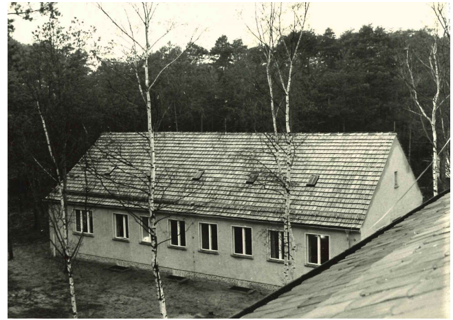
Figure 13. View from the attic floor of the main building on the electric laboratory. Source: Helmholtz Centre Potsdam – GFZ.
