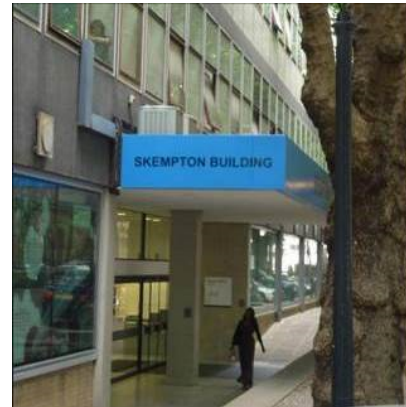
Figure 4. Imperial College. Civil Engineering Department: Skempton Building (Imperial College Web).
